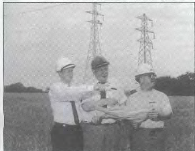
Assessing conductor profiles over adjacent roads are (l-r) CFU Line Engineer David Felton, Site Agent Len Keeble and CFU Chargehand Linesman Fred Deakin
