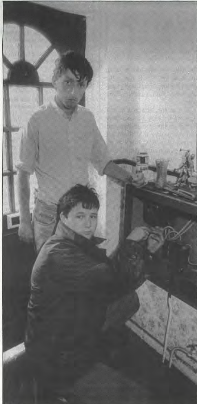
Electrician Paul Davies (front) checks fuses at flats in Conwy.
